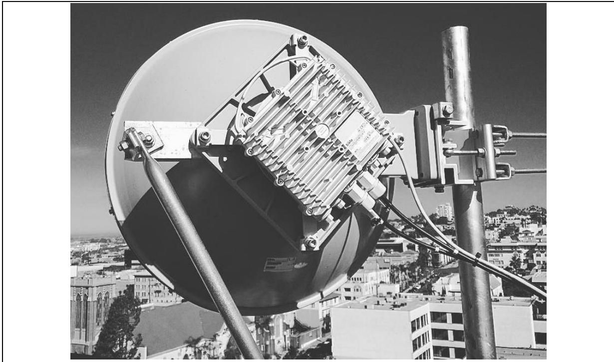
FIGURE 4a: 2FT Antenna installation (EH-ANT-2ft-B)
